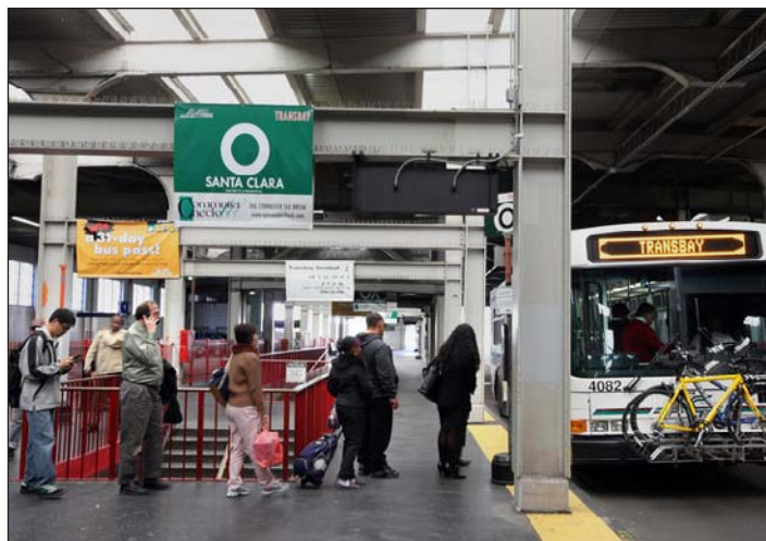
The existing transportation terminal will be demolished and replaced with the sparkling new transit center.
