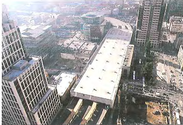
Plans are under way to redevelop the once-busy Transbay Terminal in San Francisco.
